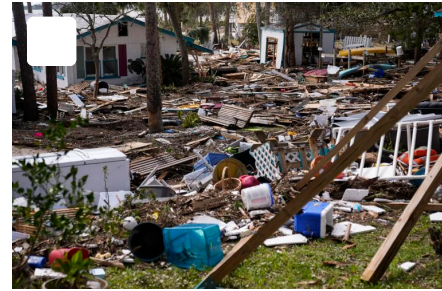
The Faraway Inn Cottages and Motel in Cedar Key, Fla. is in shambles Sept. 27 in the aftermath of Hurricane Helene.
